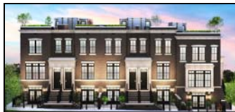
* Hargett Place Rowhomes (19 under construction)
